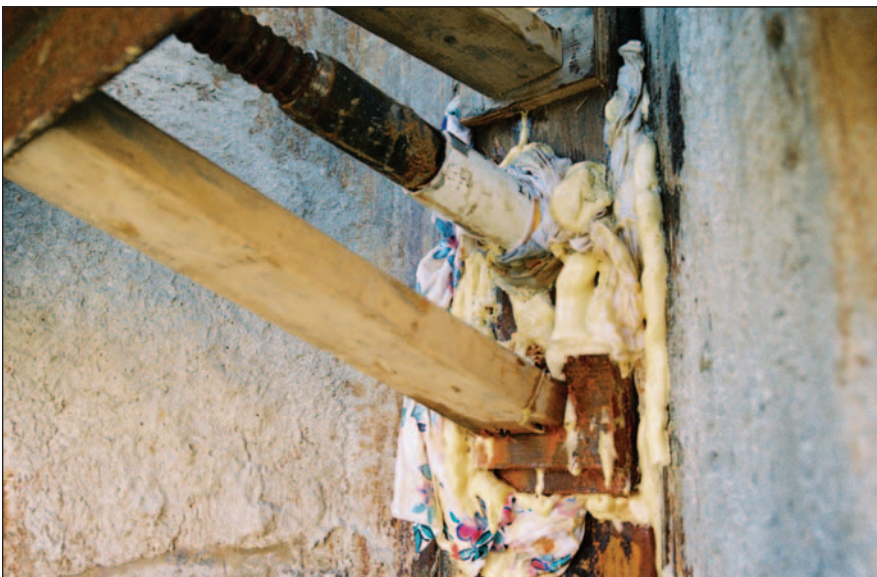
Tieback sealed with HYDRO ACTIVE® CUT
