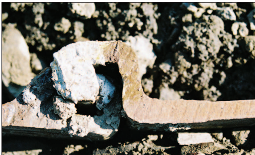
Swellseal® WA after driving sheet piles
