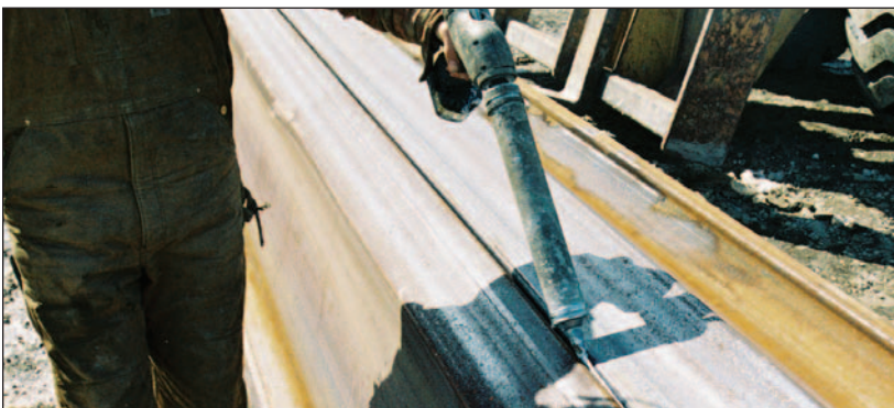
Swellseal® WA applied with caulking gun
