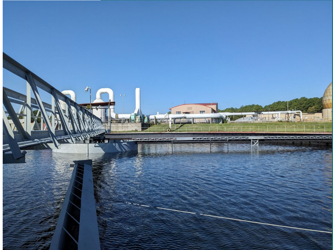
Primary Settling Tank
