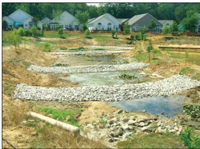
Figure 2. From 2009–2010 the town of Centerville and MDNR converted an existing stormwater management pond into a multi-cell pond-wetland complex to more effectively capture and treat runoff.
