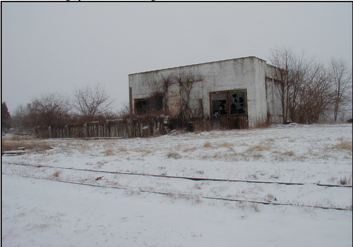
Photograph of the masonry building taken during March 6, 2001 site visit.
