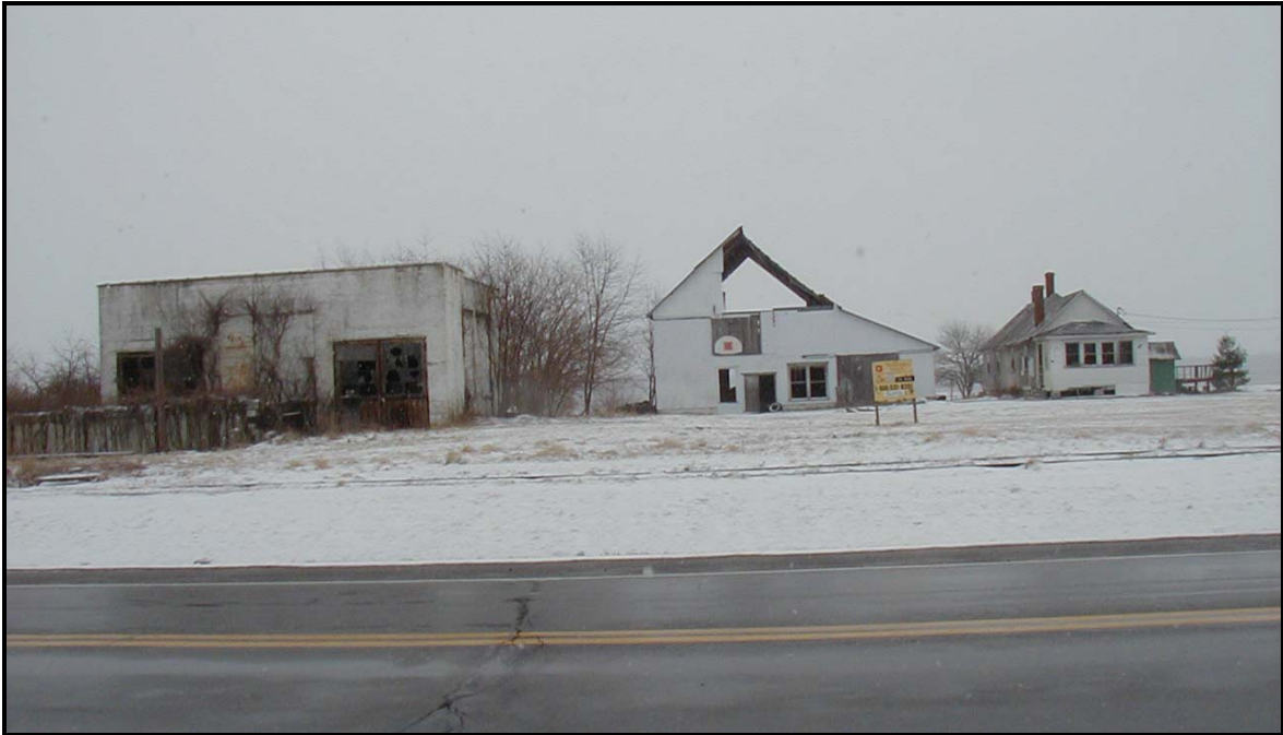
Photograph of the property and three on-site buildings from Goldsboro Road, facing southeast. Photograph was taken during the March 6, 2001 site visit.
