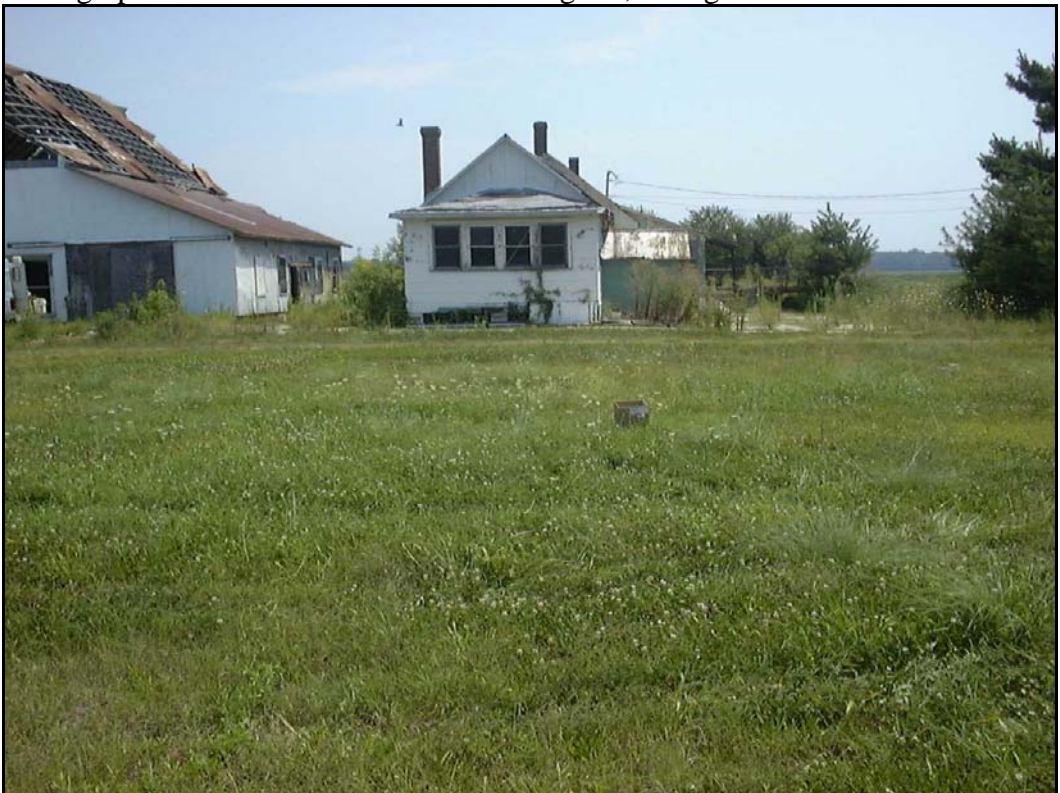
Photograph of location S-7/SS-7 facing east towards the former residence.
