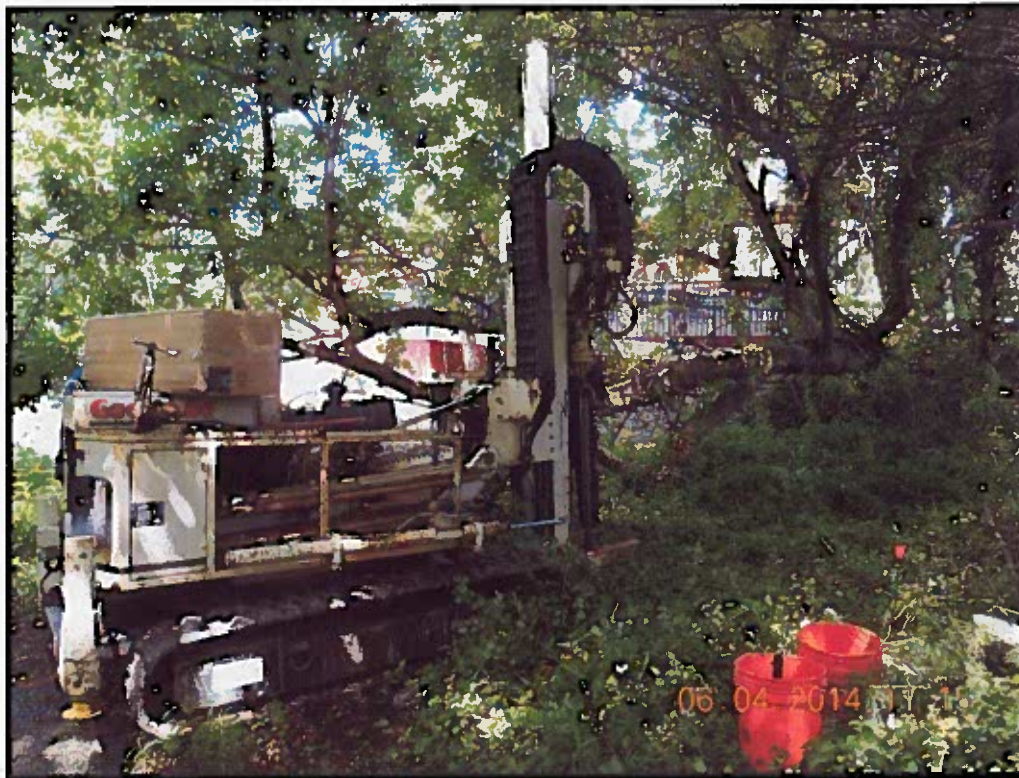
Photo 20 - S-13/SS-13 Near Site Entrance
