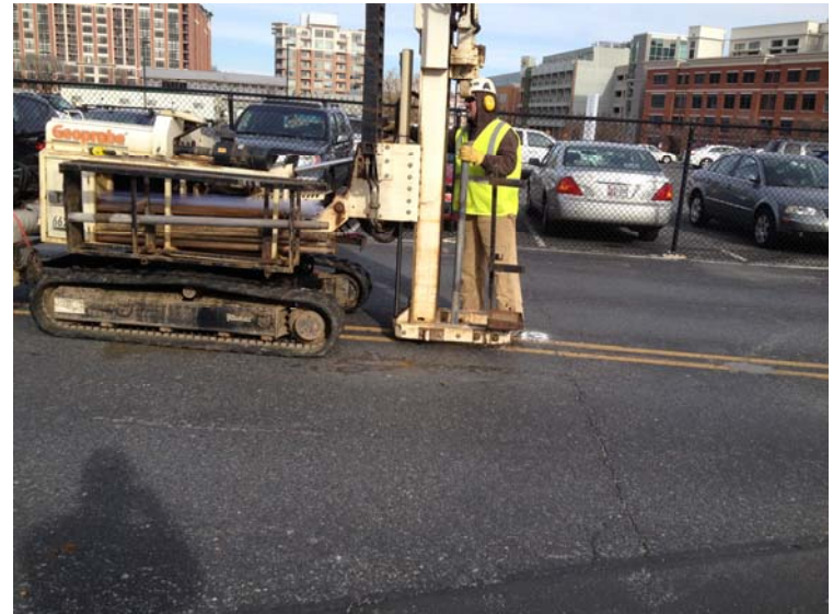
Photo 8: View of Geoprobe advancing boring GTA-13.
