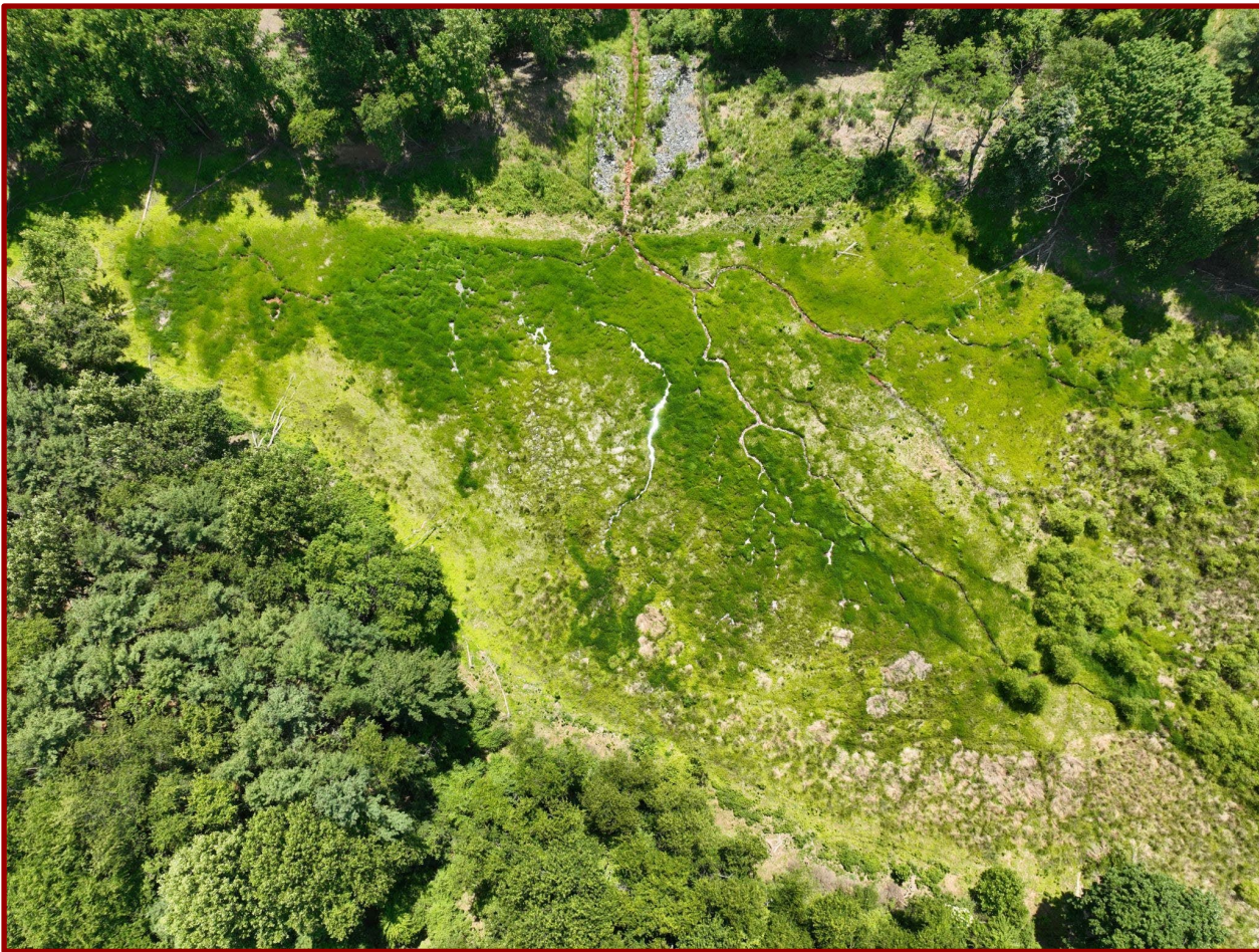
Figure 6.2: Former Martin Farm Pond Dam 54 months following breach completion.
