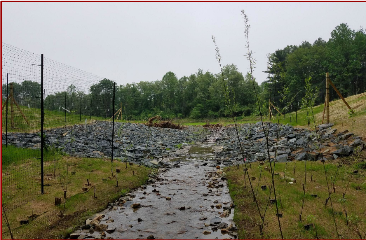
Figure 5.1: MDE photo of stabilized breach channel at former Martin Farm Pond Dam (MD Dam No. 531).
