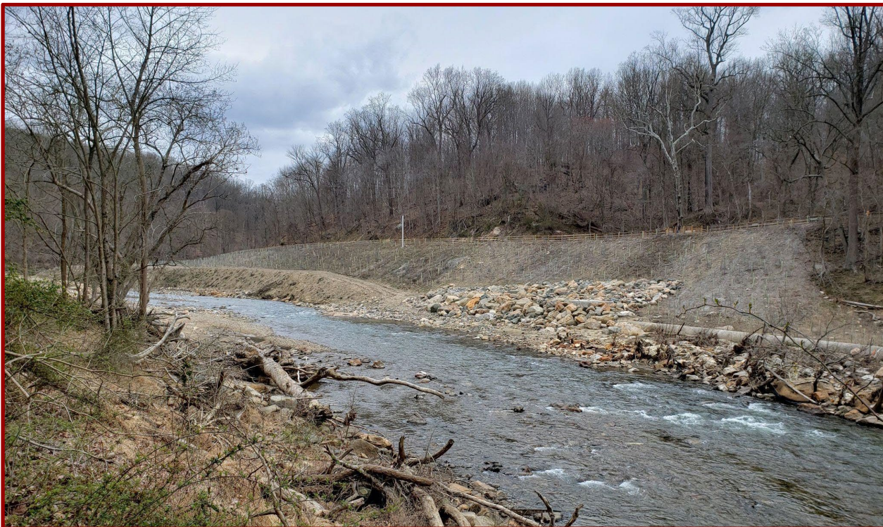
Figure 6.1: Former Bloede Dam site on the Patapsco River. Approximately 60 miles of habitat, including the mainstem and tributaries, are now open to migratory and resident fish post removal.
