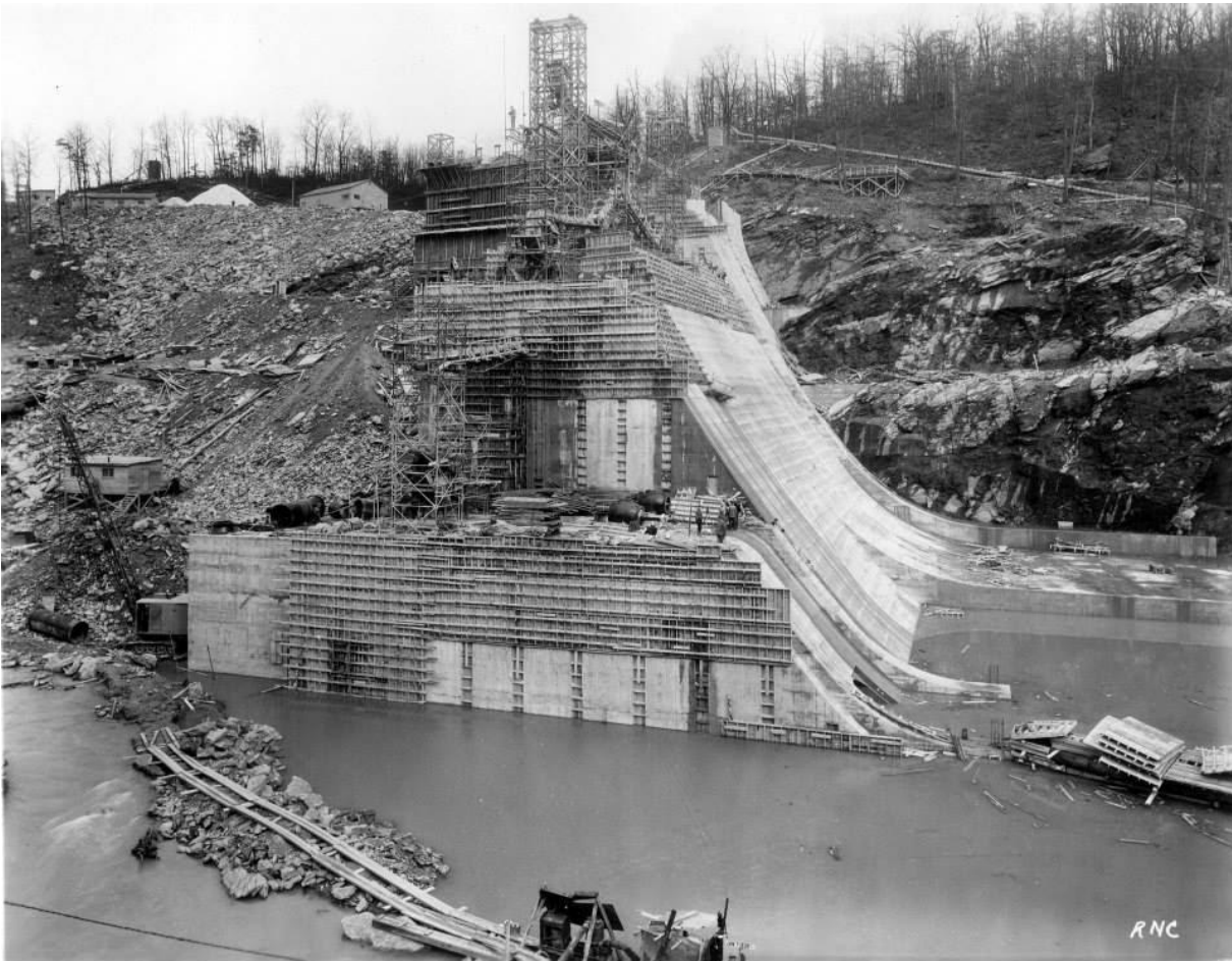
Figure 1.3: Prettyboy Dam under construction. The 7,380-acre Prettyboy Reservoir is owned by the City of Baltimore and was constructed in 1932. Image used with permission from Baltimore City DPW.
