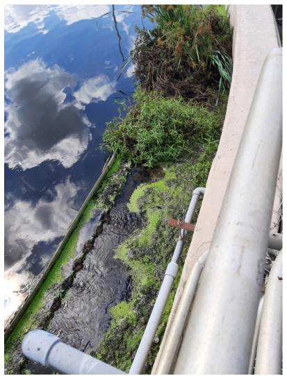
9/20/2021 Weir of secondary clarifier showing unacceptable blockage by algae and vegetative growth. This condition is impeding proper treatment process.
