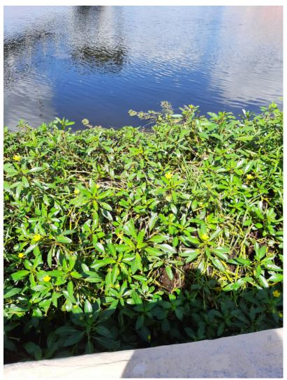
9/20/2021 In this area vegetation growth has been unchecked and allowed to grow on the weir of one of the secondary clarifiers. This condition will hinder the satisfactory treatment of the wastewater leading to poor effluent quality.
