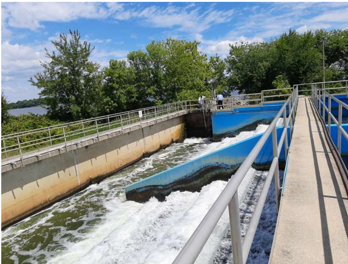
8/16/22 Final effluent at step aeration system
