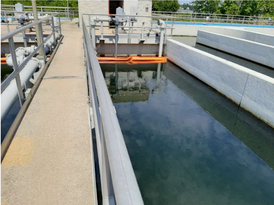
8/16/22 Recently installed booms since the last evaluation
