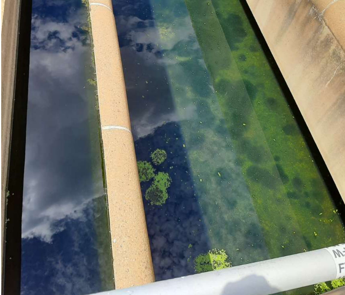
6/16/22 Quad #3 filter #11 out of service filter.
