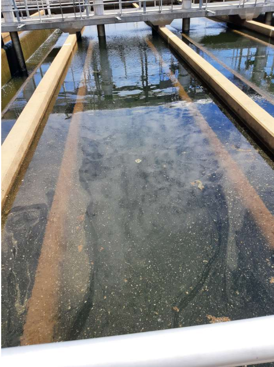
8/16/22 Submerged filter
