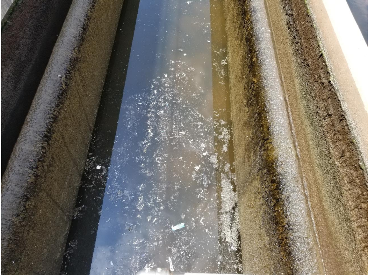
4/26/23 Solids and trash observed to be floating on water surface in the DNFs.
