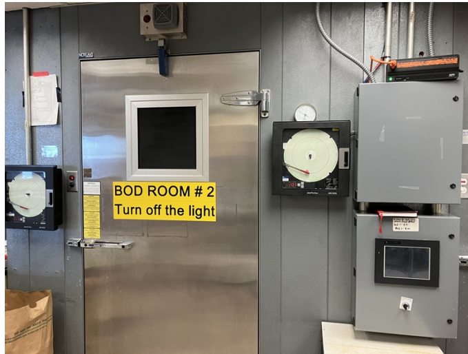
Image 3: Patapsco WWTP Lab, BOD Analysis Room
